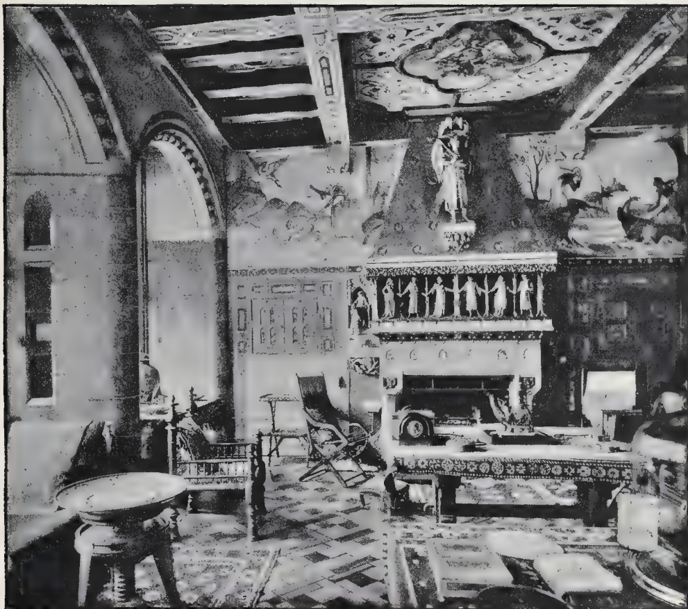
The Drawing-room of the Melbury Road House.
